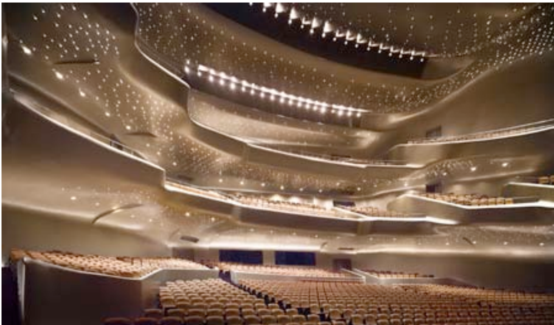
Custom molded glass-fiber reinforced gypsum (GFRC) units were used for the interior of the auditorium.
