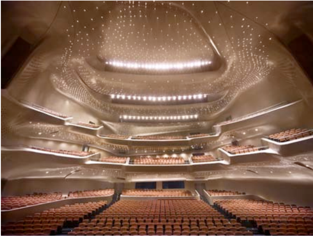
Custom molded glass-fiber reinforced gypsum (GFRC) units were used for the interior of the auditorium.
