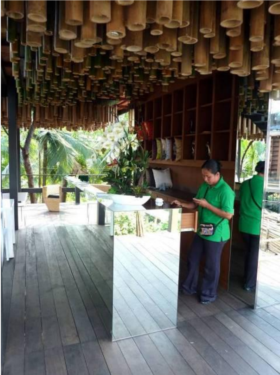
Locally sourced bamboo was used above the reception area.
