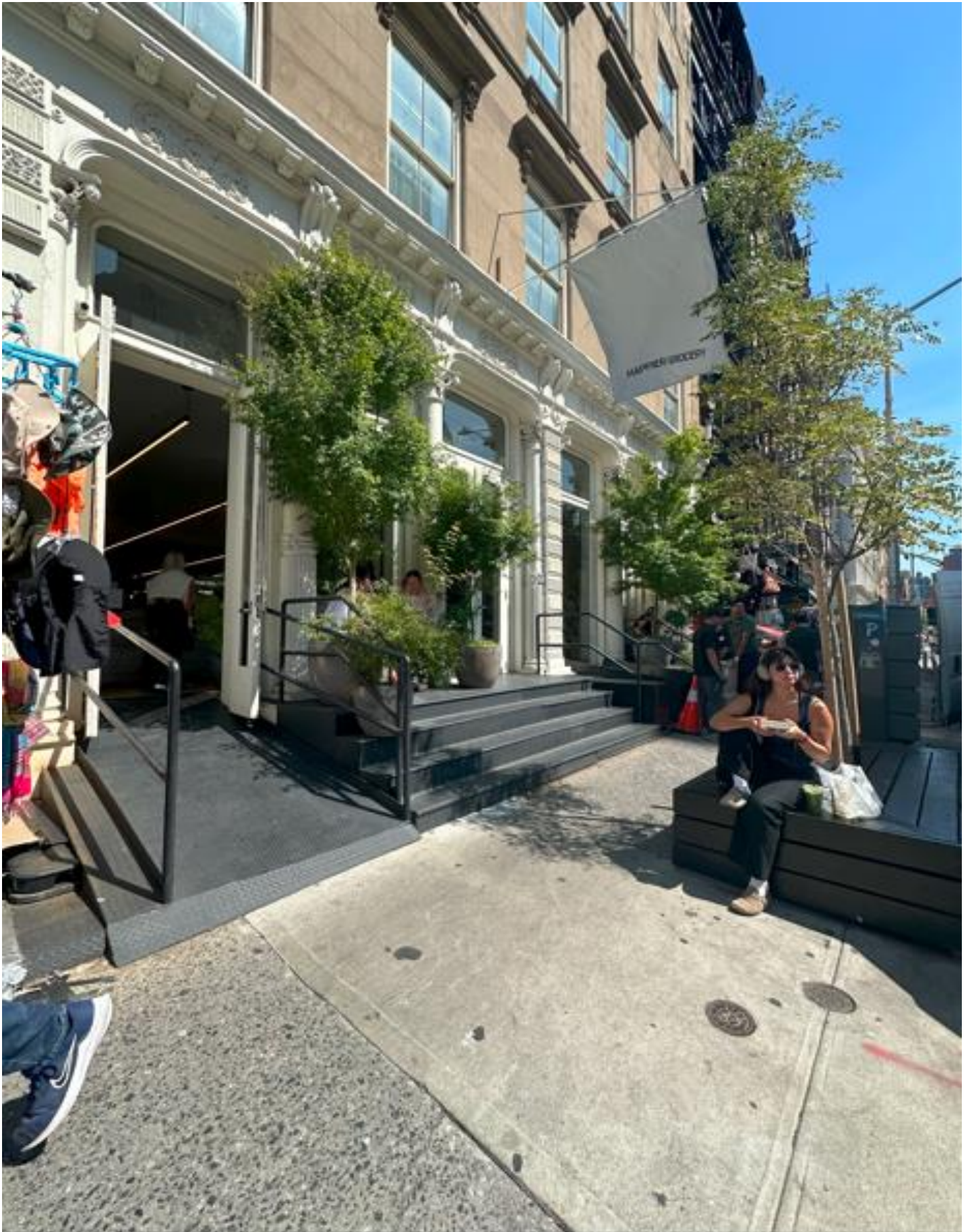
Renovation of an old building while retaining its loft-like façade
